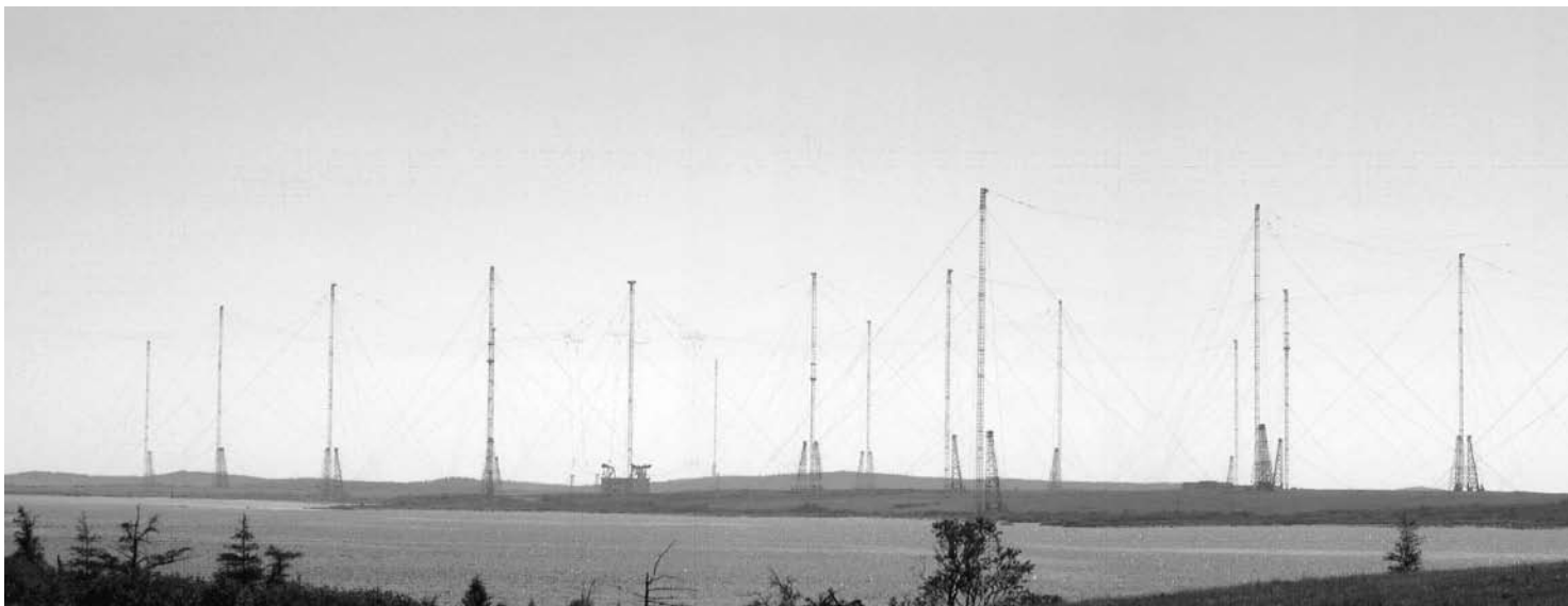
Figure 8 — Here is a photo of the antenna field for station NAA in Cutler, Maine.
